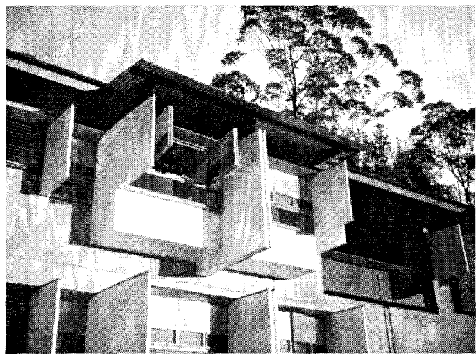
Figs. 1 & 2. Window and shade assembly of a typical sleeping quarter. Riversdale Educational Retreat Center, Bundannon, New South Wales, by Glenn Murcutt with Reg Lark and Wendy Lewin, 1999.
